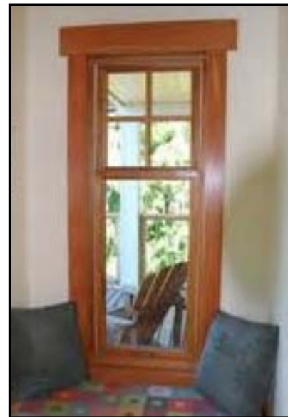
Put window casings around a window
