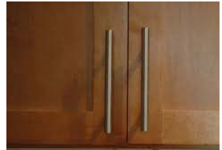
Overlay: None of the cabinet face-frame is seen
