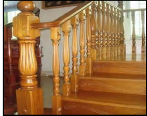
Stairs and balusters
