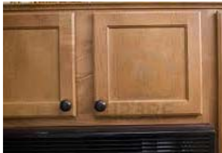
Lipped: Part of the cabinet face-frame is seen
