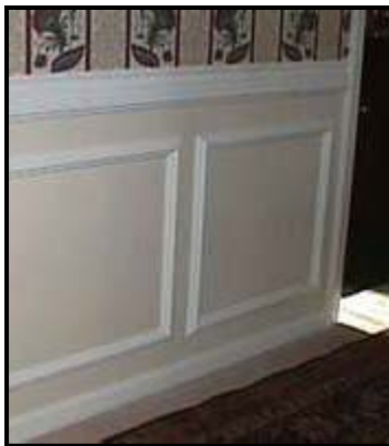
Attach a chair rail or wainscot
